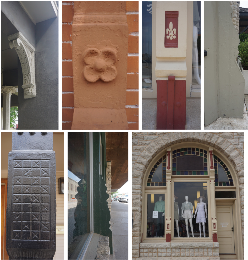
The small details found on buildings throughout Downtown subtly contribute to Stephenville’s charm and identity. Some of these details include wood carvings, stained glass, ironwork, masonry carving, and brickmaker stamps.
