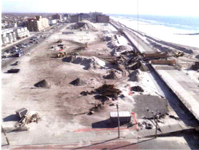
Sand Reclamation and Screening Site
