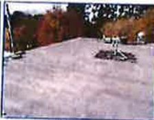
Flat roof view
