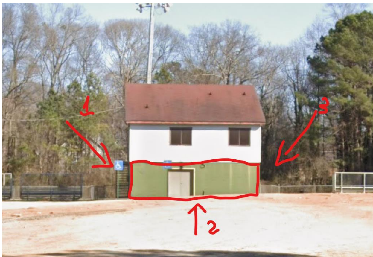
3 walls of the concession stand (the main wall facing the parking lot, and the two walls around).
