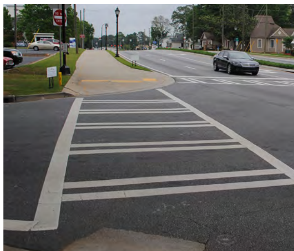
High-Visibility Crosswalk with Pedestrian Countdown Signal, Cobb County, GA
