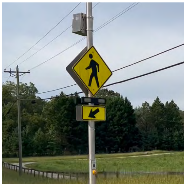
Rectangular Rapid-Flashing Beacon on Klondike Road Near Vaughter's Farm Trailhead
