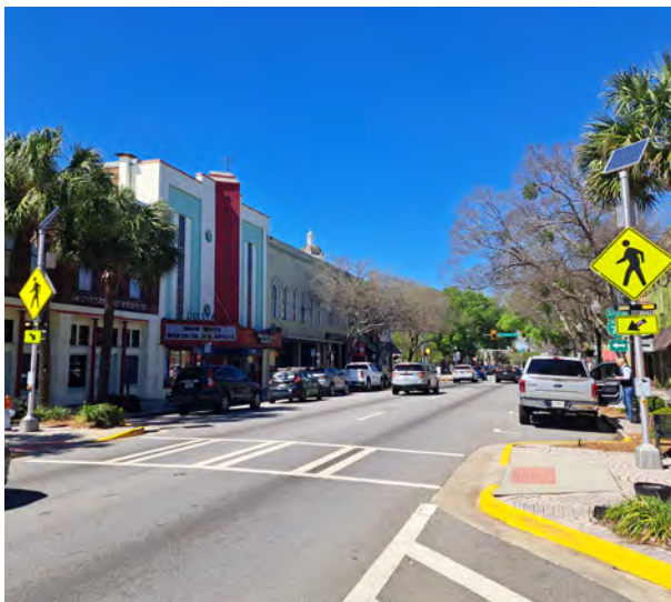
Rectangular Rapid Flashing Beacon, Valdosta, GA
