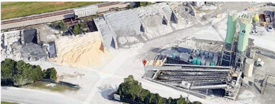
Exemplar: ready-mix concrete batch plant
