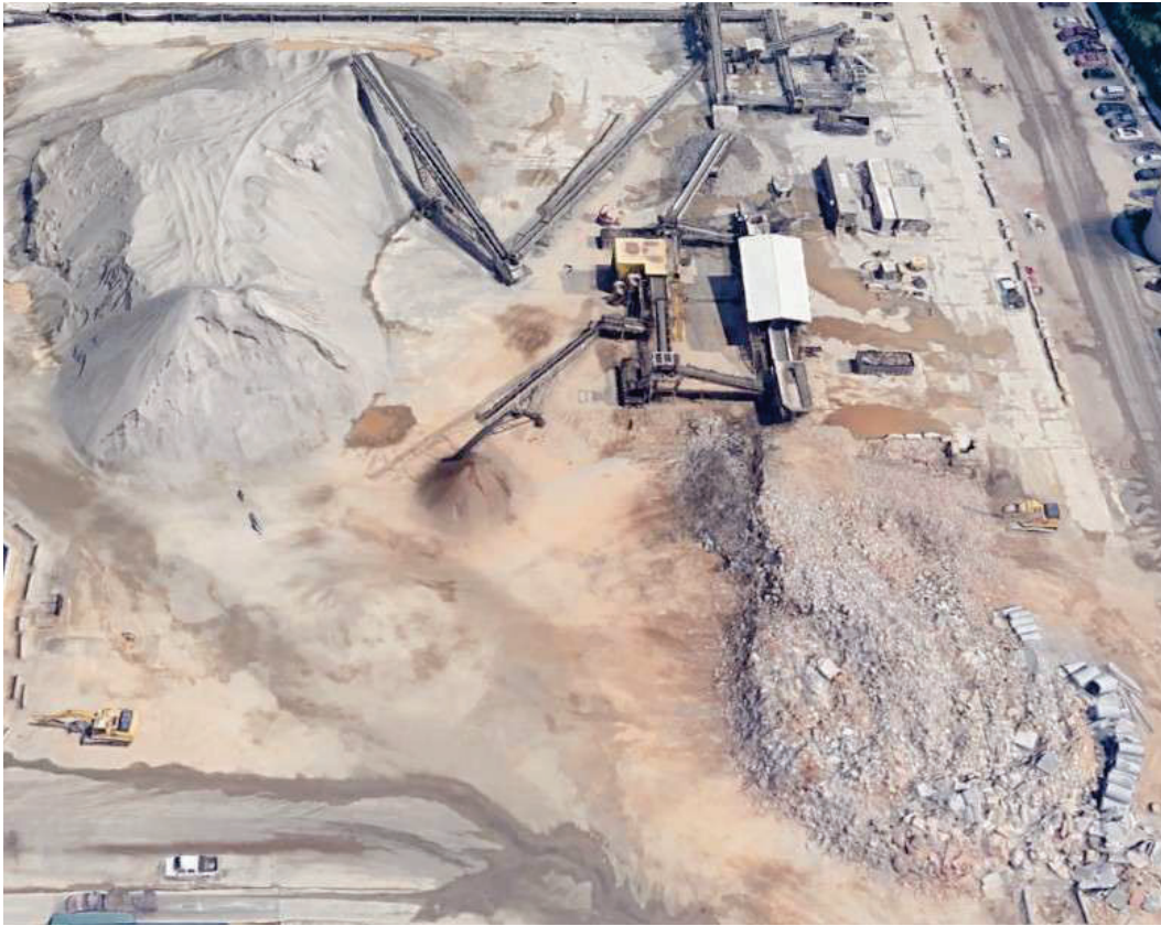
Exemplar: MetroGreen Pleasantdale concrete recycling facility
