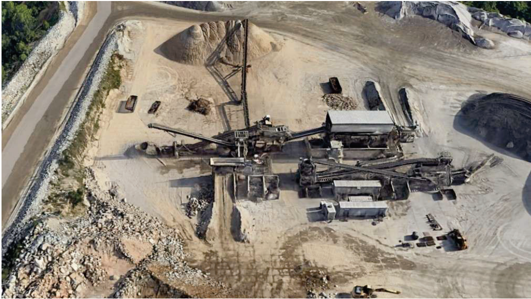
Exemplar: asphalt production plant
