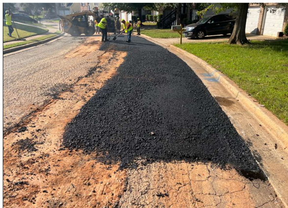
Roads with most the base and subbase missing.
