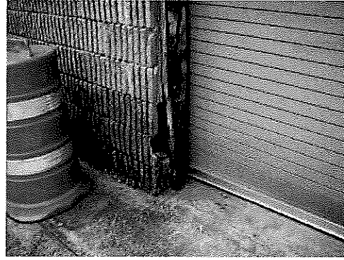
Repair CMU Wall
