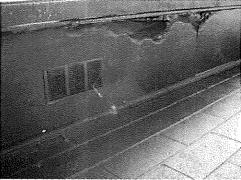
Soffit at Rear of Building
