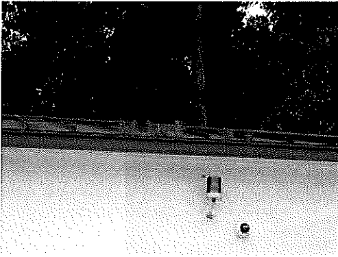
Gutter at Lazy River Pump Room
