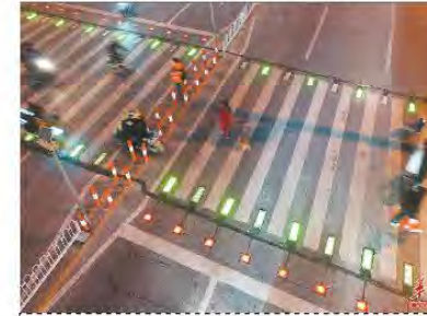
Signalized trail crossings
