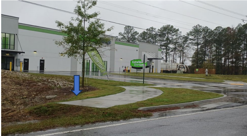
Photo at left accurately shows the start of the new sidewalk in front of existing storage facility
