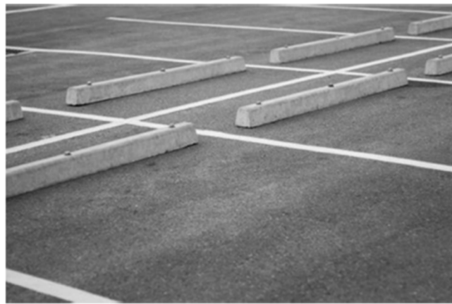
Wheel stop placement in "head-to-head" parking layout
