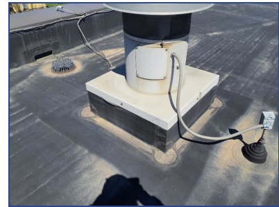
Membrane Shrinkage
