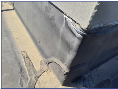
Membrane Shrinkage
