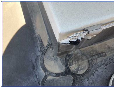
Membrane Shrinkage
