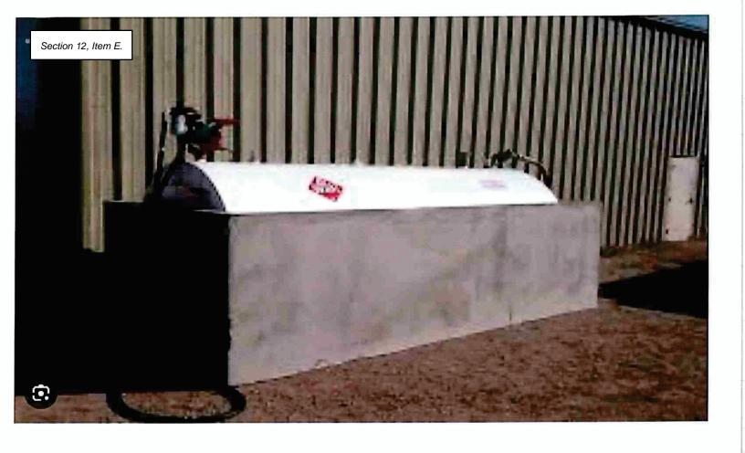
This is what the spill containment looks like with the tank inside of it which is large enough to hold the spilled fuel in the unlikely event of a spill, I would also like to put a roof over the top of the tank.
