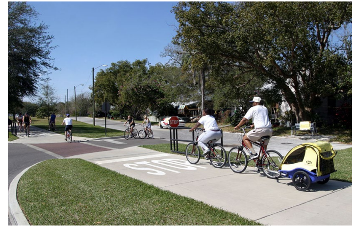
Shared Use Path (also called a paved multiuse trail, some may also be a side path)
