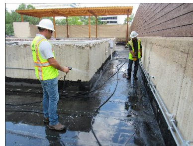
Walker employees performing ELD on hot rubberized asphalt waterproofing
