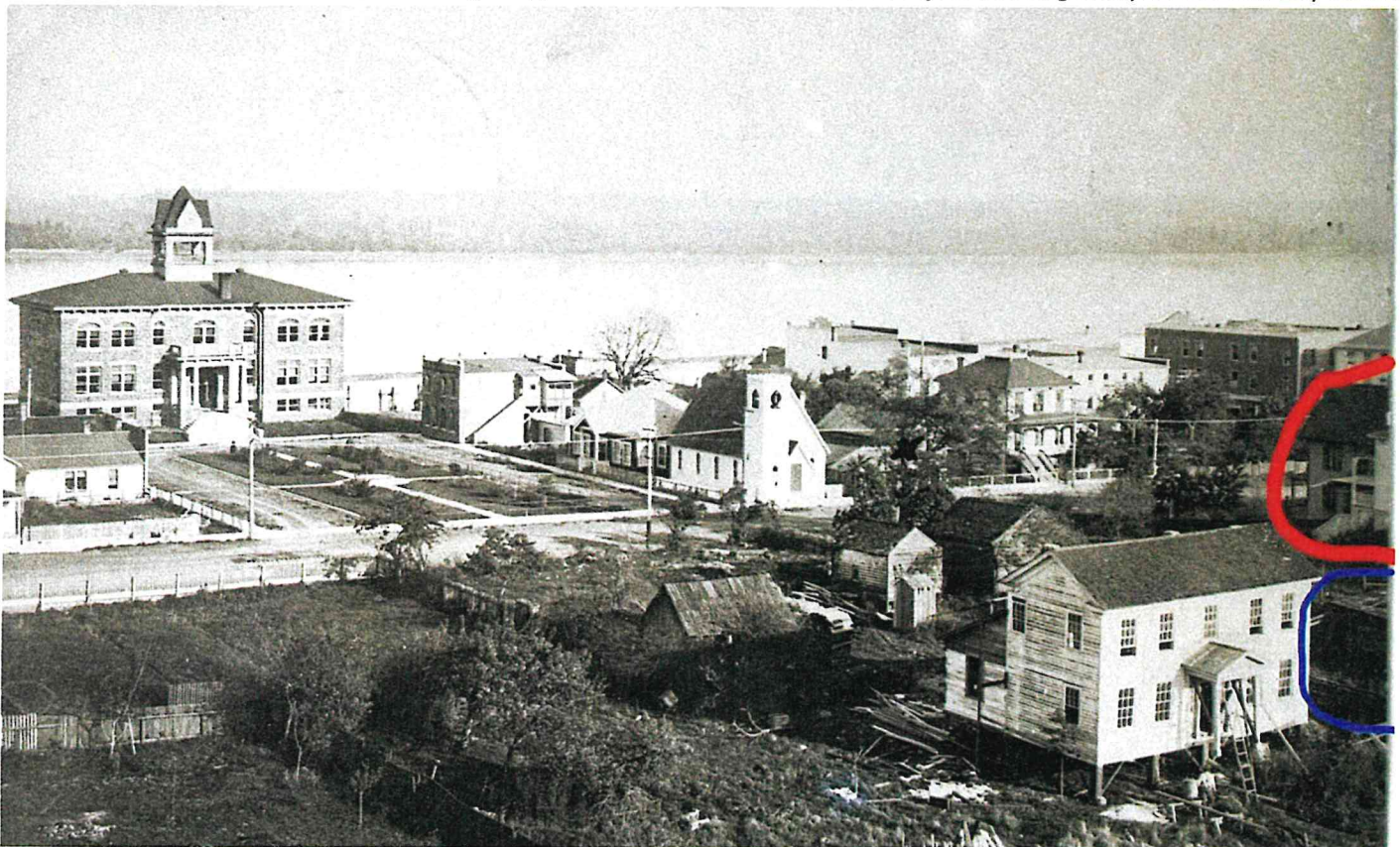
1912-1915 - The 2 nd location of the Henry Knighton House shown in the foreground. The subject dwelling can be seen in red. CCMA believes the location of the barn being deconstructed may be in circled in blue. Photo courtesy CCMA.
