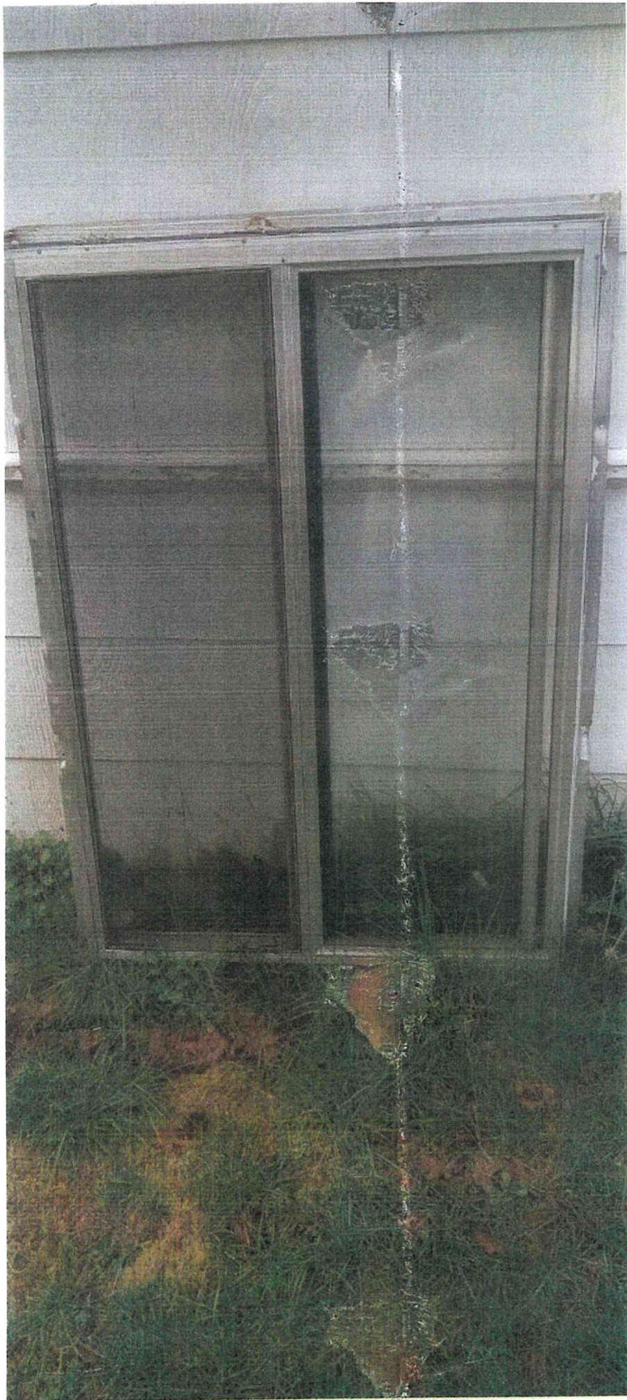
Aluminum Window Removed From North Elevation
