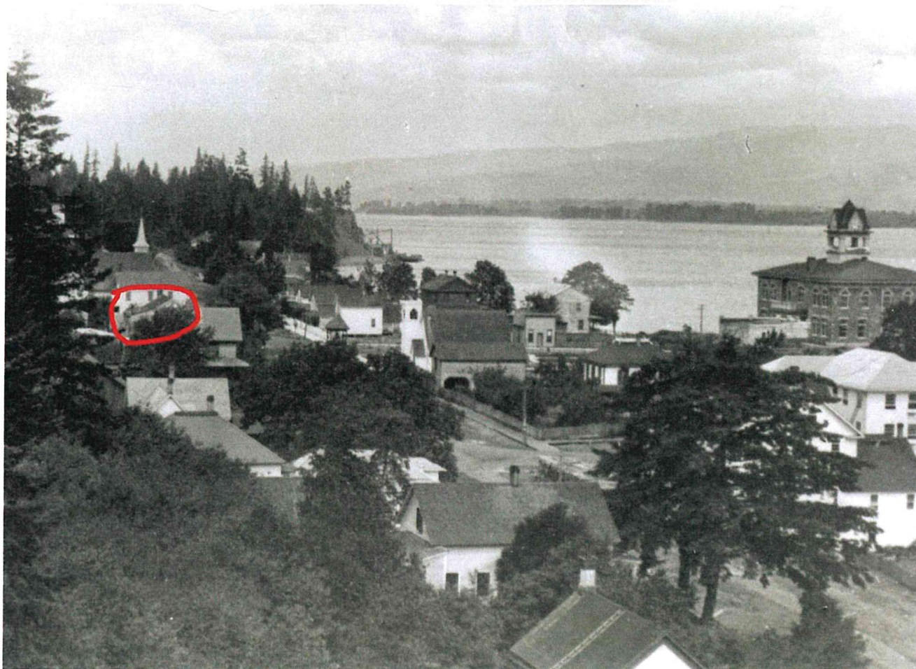
1909 - This appears to be the oldest photo of the structure. Photo courtesy CCMA.
