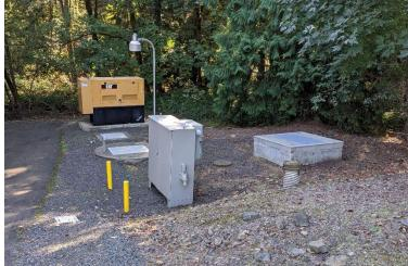
were to overflow, it would overflow at the wetwell lid and onto the site. The station is reported to have high I/I, with City staff confirming that it is normal to have an overflow event once every two years. Additionally, it was reported that a high amount of non-flushable items tend to accumulate in the wetwell, resulting in City staff needing to use a vacuum truck to empty the contents out of the wetwell approximately once every quarter.
