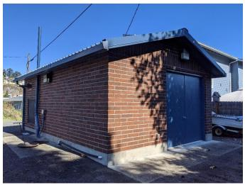
building. There is no fall protection installed at the pump station.
