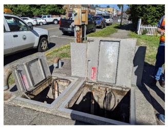
opened manually. The level is recorded via an ultrasonic level sensor with backup floats, however there is no fall protection installed at the pump station.
