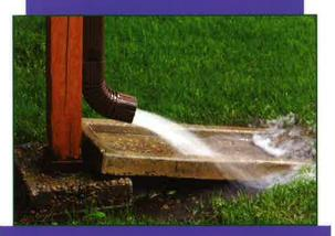
In wet weather it only takes a few improperly connected sump pumps to cause a sanitary sewer backup into basements, streets and waterways. Page 500
