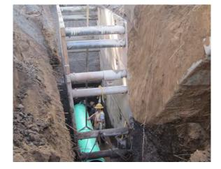
Consor provided complete engineering services to the City of Springfield for the Jasper Road Trunk Sewer project. Services included detailed alternatives analysis, design, bidding and construction management. The project consisted of approximately 20,000 feet of new gravity trunk sewer ranging from 12 to 27 inches in diameter.
