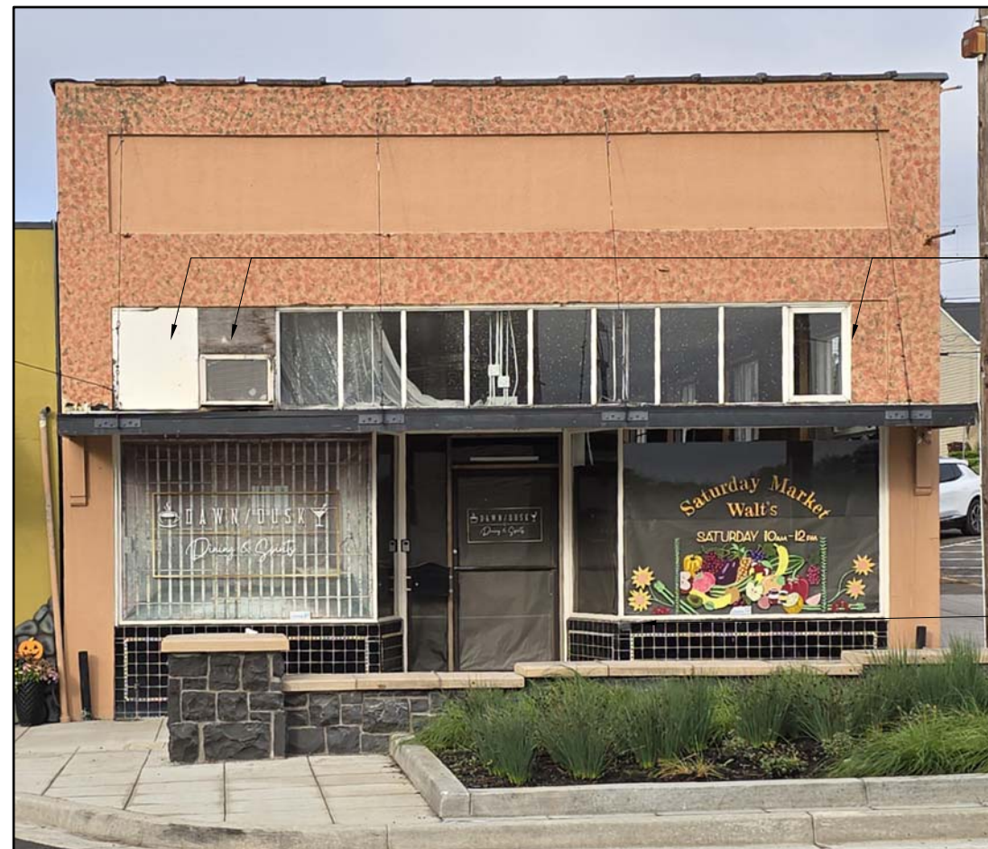
REMOVE HVAC UNIT, REPAIR WD WINDOW FRAMES & GLAZE WHERE REQUIRED
