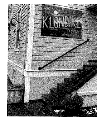
Porch and stair siding to match Existing vertical skirt siding And 1x6" trim.
