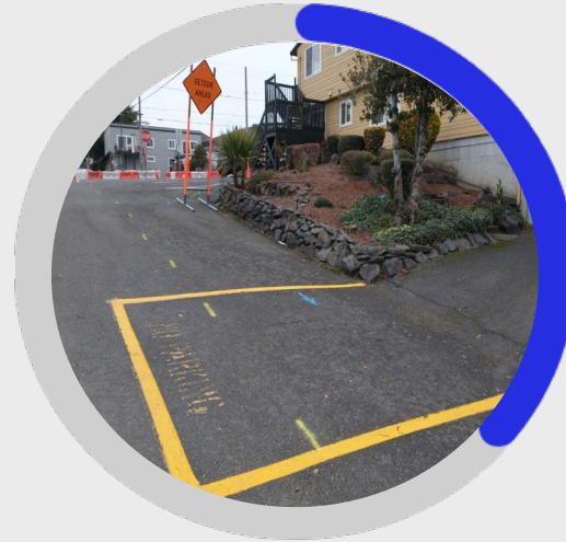
S 1 st St/St. Helens St Undergrounding
