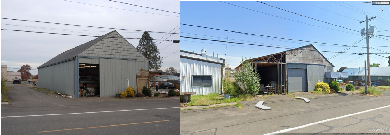
Left Photo: February 10, 2014 of 184 S. 15 th Street before the proposed building addition. Right Photo: Google Earth street view May 2023 long after the building addition project had been abandoned and permits expired, but landscaping was still intact, including the area between the building and sidewalk. This shows a driveway along the north side of the building that was eliminated with the building addition.
