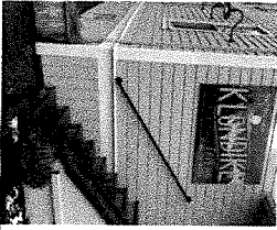
Porch and stair siding to match Existing vertical skirt siding And 1x6" trim.
