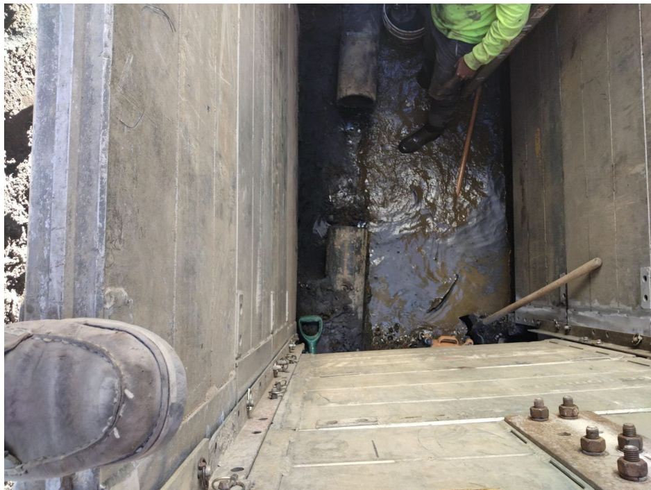
Contractor replacing 4 ft section of 8 in underground pipe, approx. 10 ft down. Coffor walls installed and continuous air monitoring conducted to ensure worker safety during the repair.
