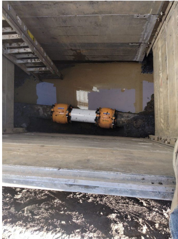
New 4 ft section of pipe installed to repair leak on 8/1/23. Line tested. No leaks.
