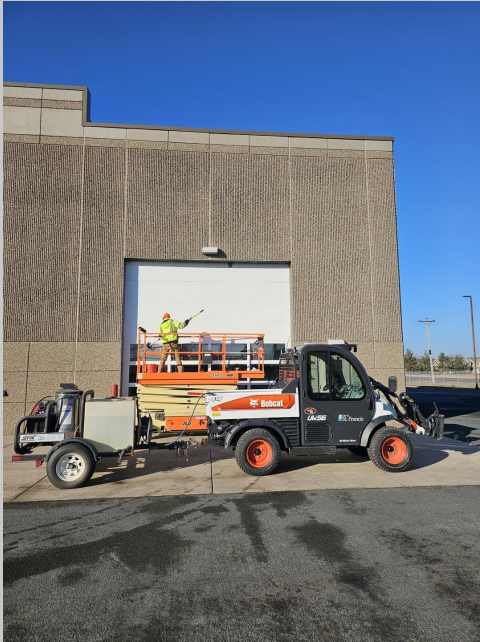
Cleaning grease and dirt off garage doors.
