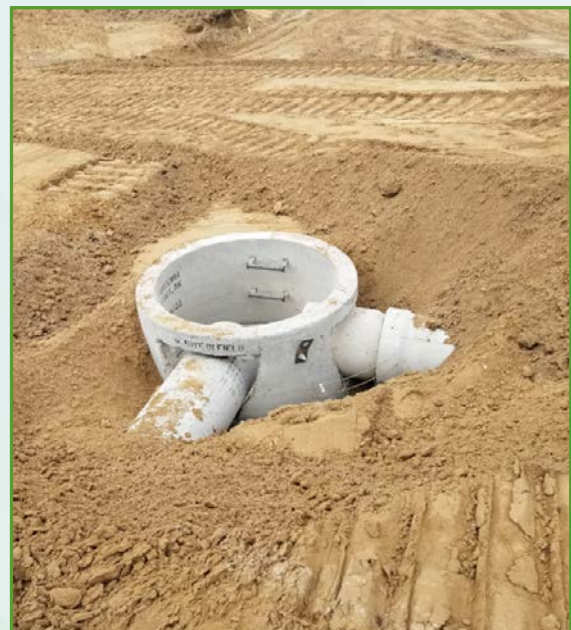
Siwek Park storm sewer installation.
