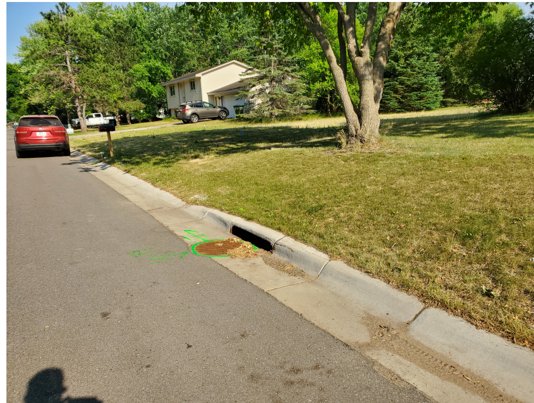
SITE OVERVIEW FACING SOUTHEAST, CATCH BASIN IN FOREGROUND
