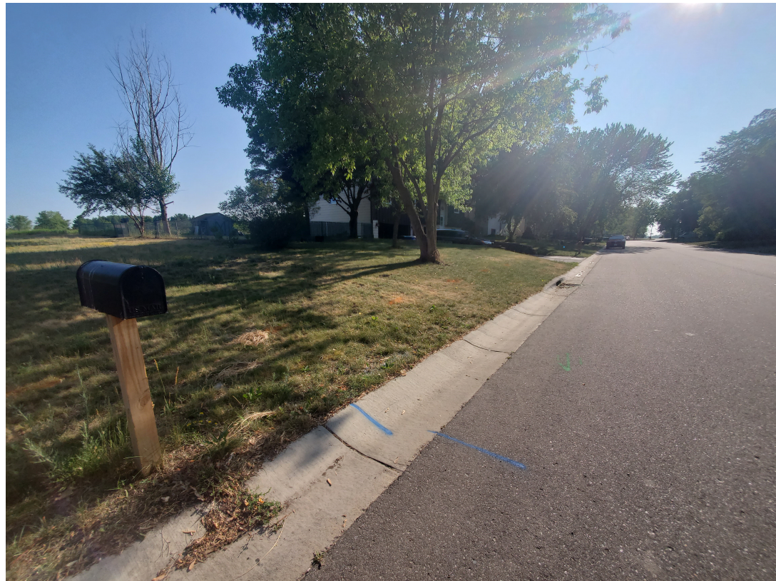
SITE OVERVIEW FACING SOUTHWEST, CATCH BASIN IN BACKGROUND
