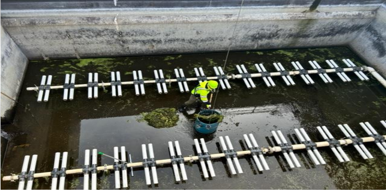
This is what the membranes look before installation. Essentially, they are perforated rubber that diffuses the air supply allowing for a uniform treatment.
