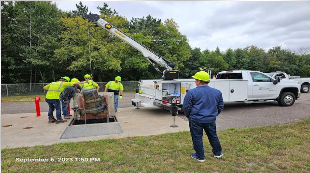
Our new crane truck arrived and by all accounts, has not disappointed! The picture above is a staff training session and putting it to the test, pulling our largest pump. And it passed with flying colors!
