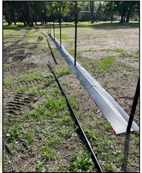
Underfencing installation to prevent grass from growing up between the fence.
