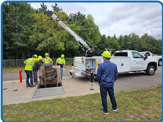
Staff cleaning out the aeration basin and prepping for membrane replacement. First step is to clean the basin. After that, staff removed the old and installed new membranes.
