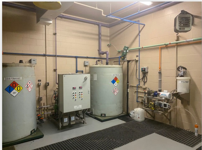
Sodium Permanganate Tanks
