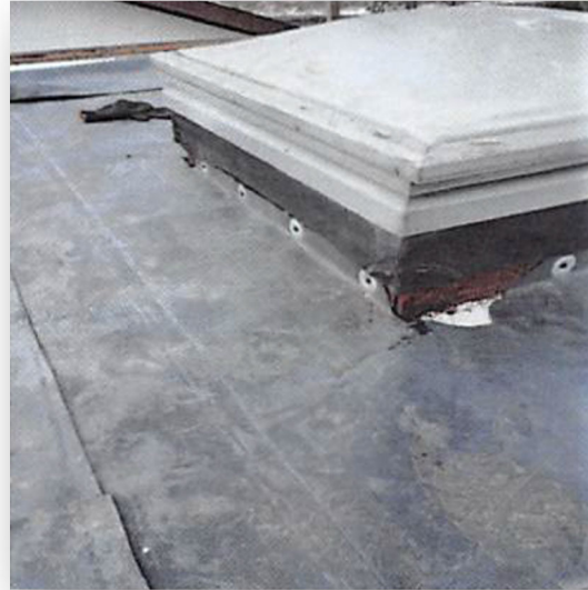
Membrane failing along the skylight
