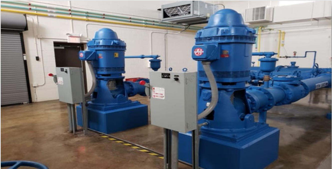
Water Treatment Facility High Service Pumps
