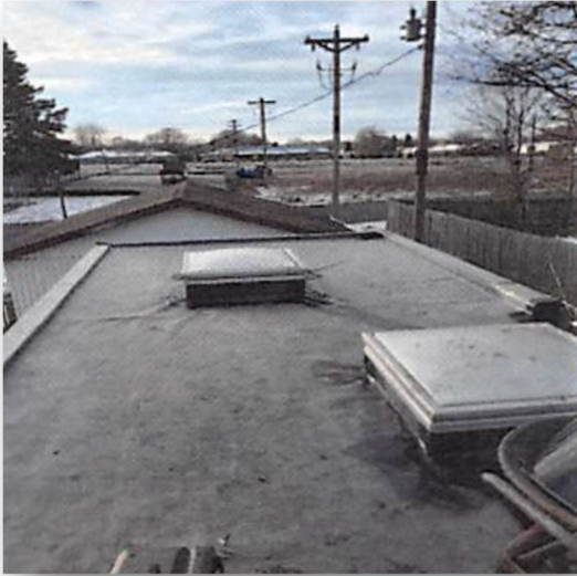
New membrane installed
