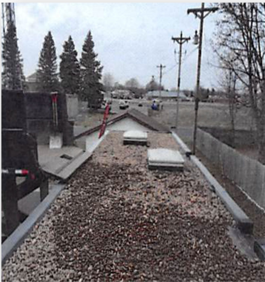
New ballasted roof complete
