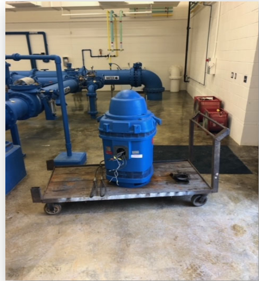
High Service Pump #1 Motor
