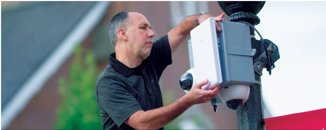
Using cellular modems, the City of Parkersburg has deployed 10+ cameras in remote locations to increase coverage where a typical network connection wouldn't be available, all without sacrificing image quality or reliability due to Verkada's onboard storage.
