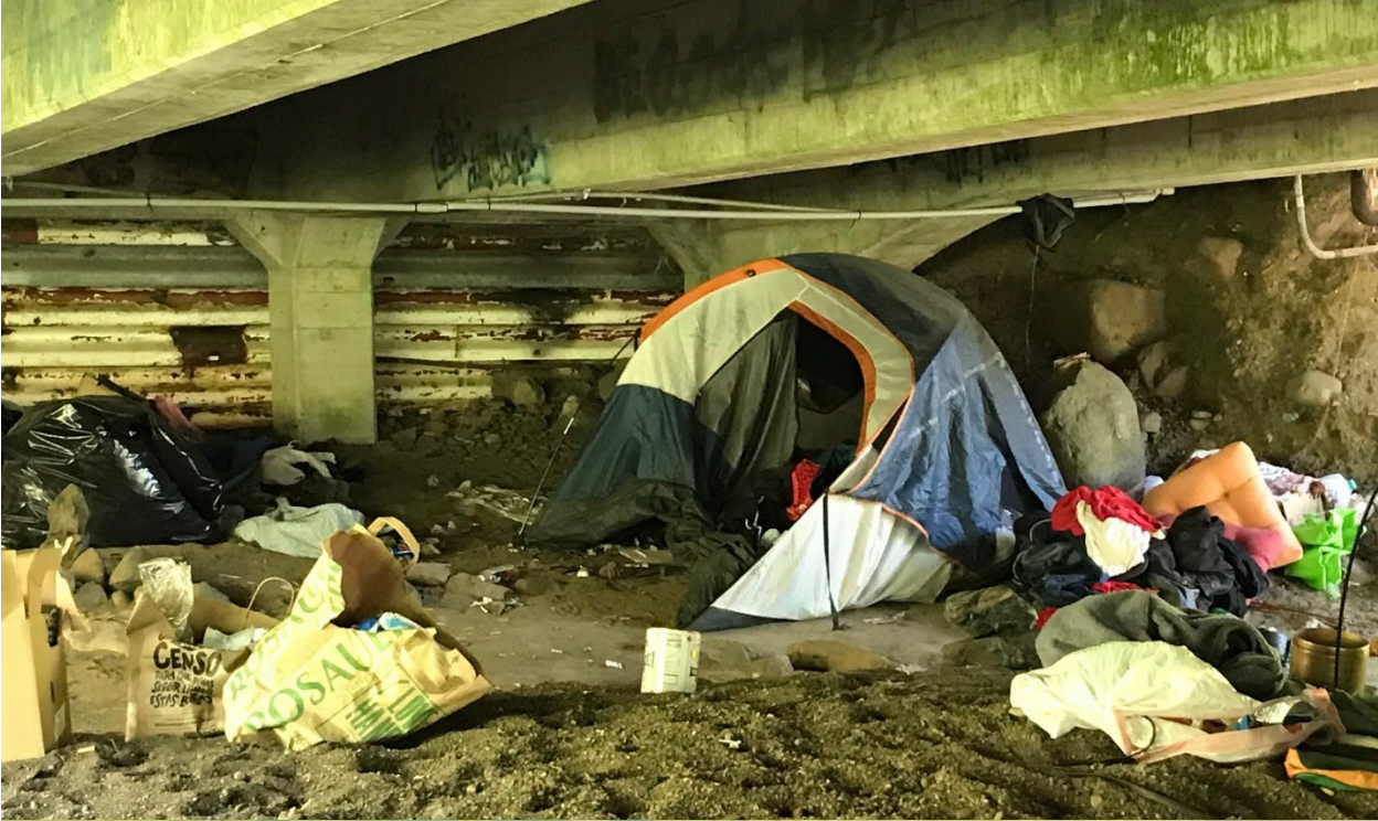
Same encampment under Rock Creek Bridge on 7/26/21.
