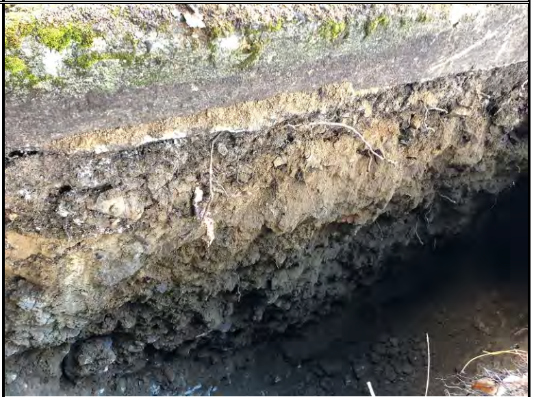
Exposed subsurface soil profile within test-pit TP-6
