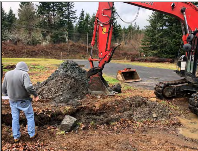
Excavation of test-pit TP-1, looking west
