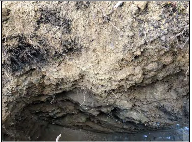
Exposed subsurface soil profile within test-pit TP-5
