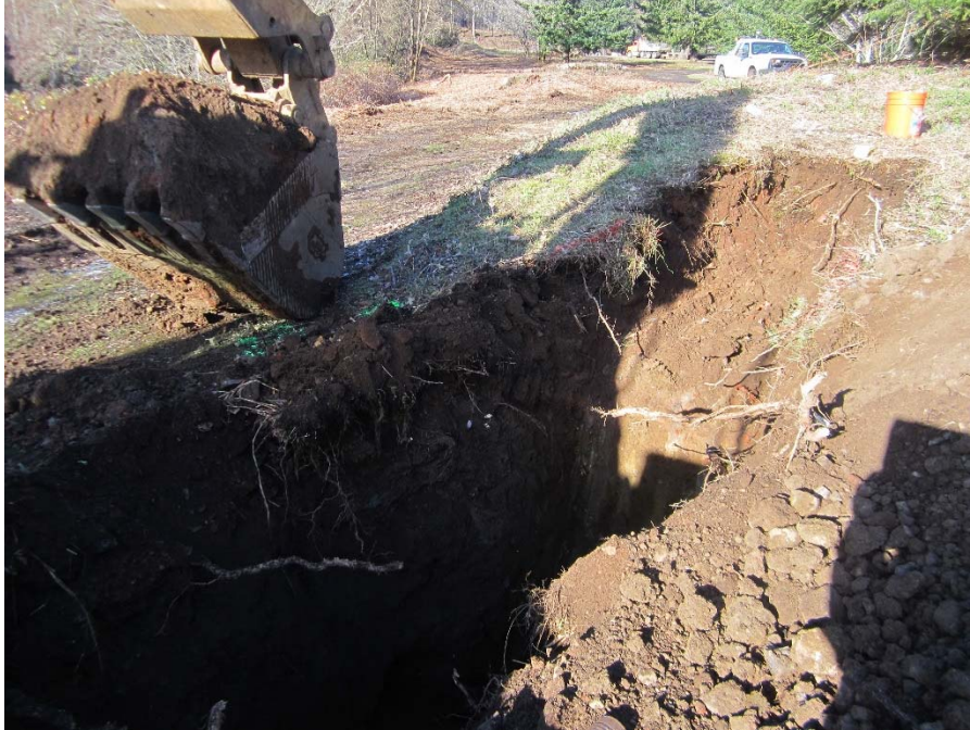
Photograph 5: Excavation of TP6 within the footprint of the southern former wigwam burner. The shelf feature in the photograph is a concrete slab encountered during advancement of the test pit. Photograph taken facing northwest.
