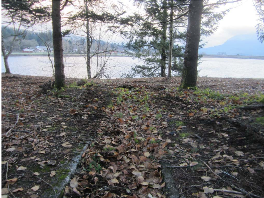
Photograph 1: Trench feature that crosses the northern part of the large building foundation. Photograph taken facing east.
