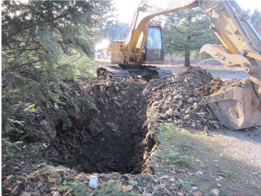
Photograph 7: Excavation TP9, which had angular cobble fill from surface to approximately 5 feet below ground surface. Photograph taken facing south.
