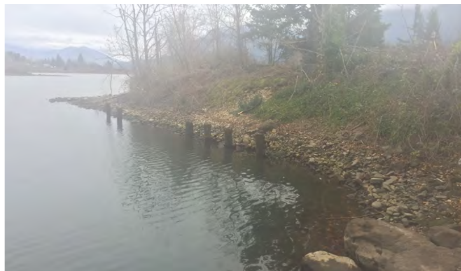
Photo 4. Riprap on the eastern shoreline, facing south.
