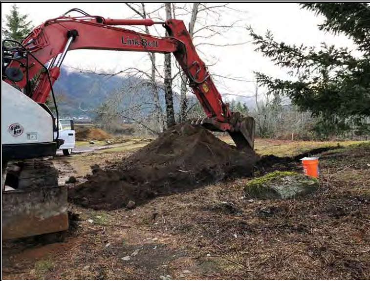
Exposed subsurface soil profile within test-pit TP-11
