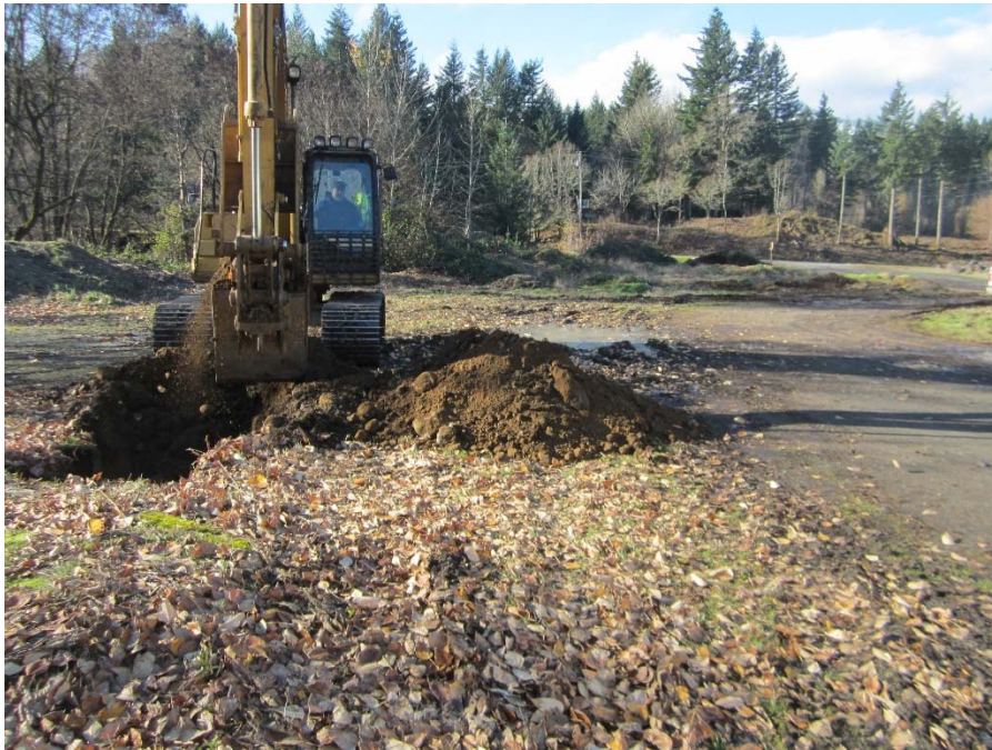
Photograph 6: Excavation TP8 adjacent to the northeast corner of the small structure foundation. Photograph taken facing west.
