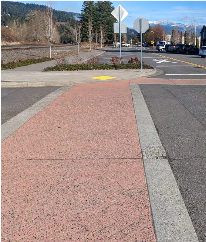
Existing crosswalk improvements for pedestrians.
