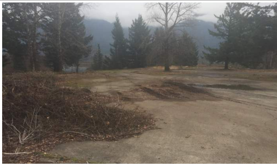
Photo 1. Existing concrete and gravel surfacing.
