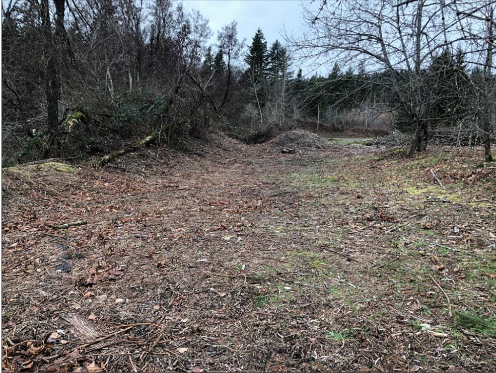
Figure 4. Photographic overview looking north of an area cleared of brush. The vegetation and displaced soil have been pushed into low piles.
