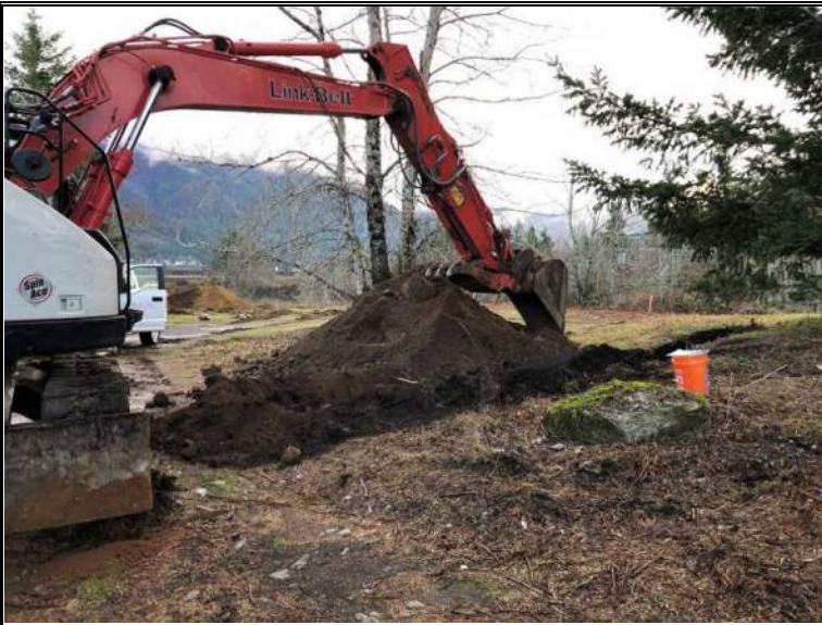
Exposed subsurface soil profile within test-pit TP-11
