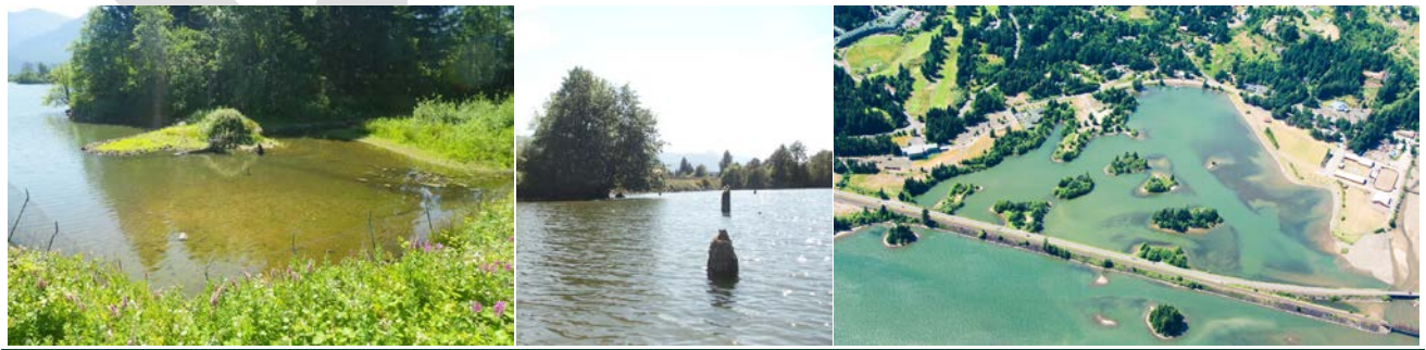
Rock Cove Degradation & Restoration Opportunities Pilings, fences, & dredge basins provide visible relics of Rock Cove's industrial past.
