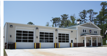
A7 Roanoke Island Fire Department
