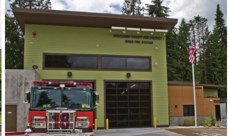
A5 Snohomish County Fire Station 18 - TCA
