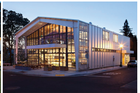
SHED - Jensen Architects B8
