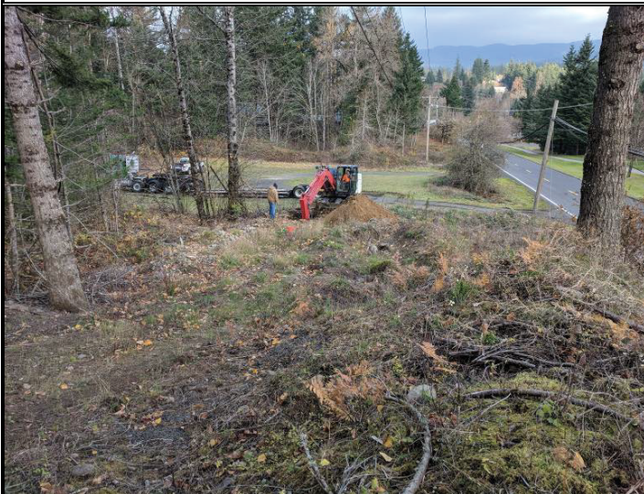
Excavation of test-pit TP-1 looking north
