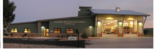
Montrose Fire Protection District Station 2 B6
