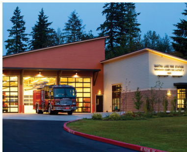
Snohomish County Fire Station 21 - TCA B7
