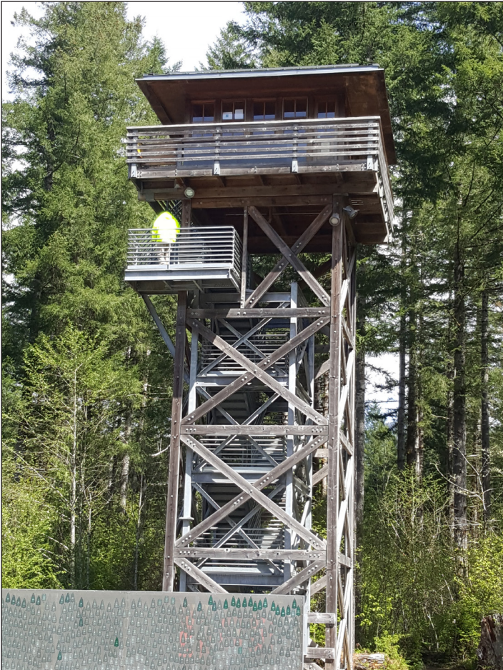
Potential Phase II Interpretive Center similar to the Tillamook Center shown here.
