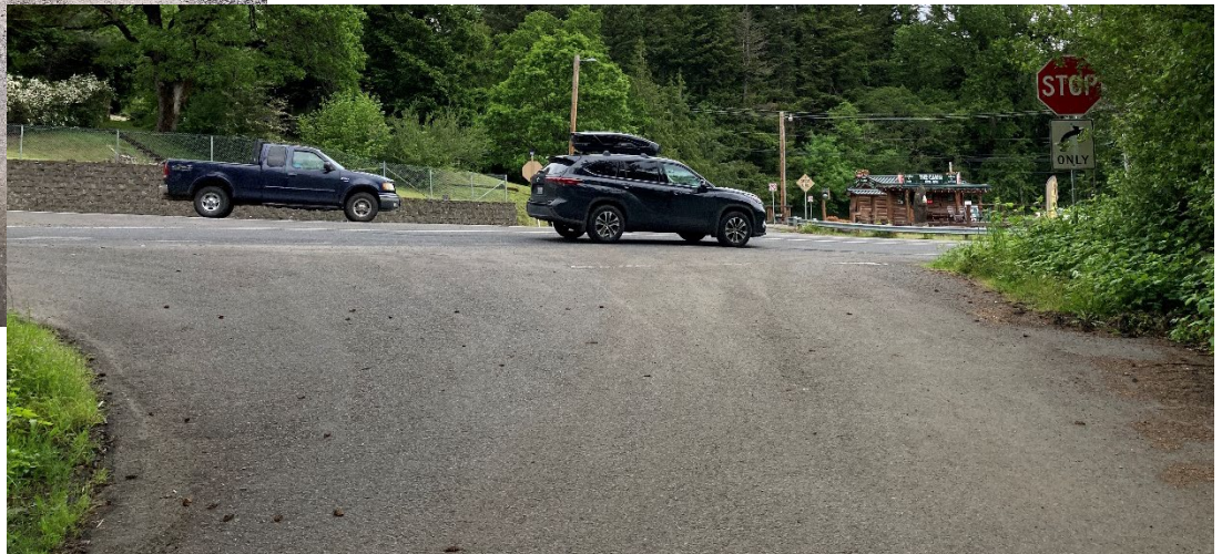
Below-View from Kanaka Creek Underpass of the intersection with SR-14.
