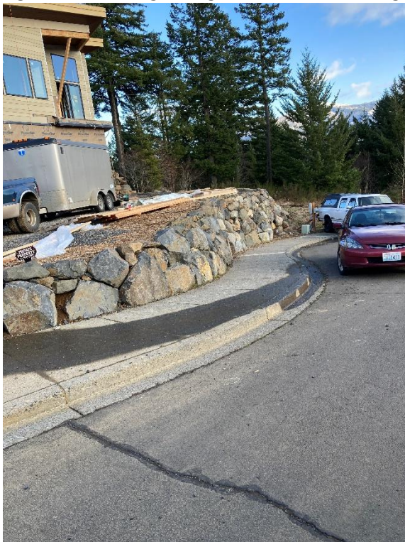
Figure 3 – 725 Angel Heights Rock Wall Looking South
