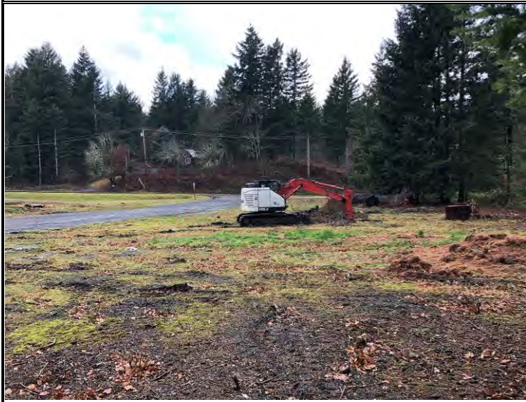
Excavation of test-pit TP-3, looking west
