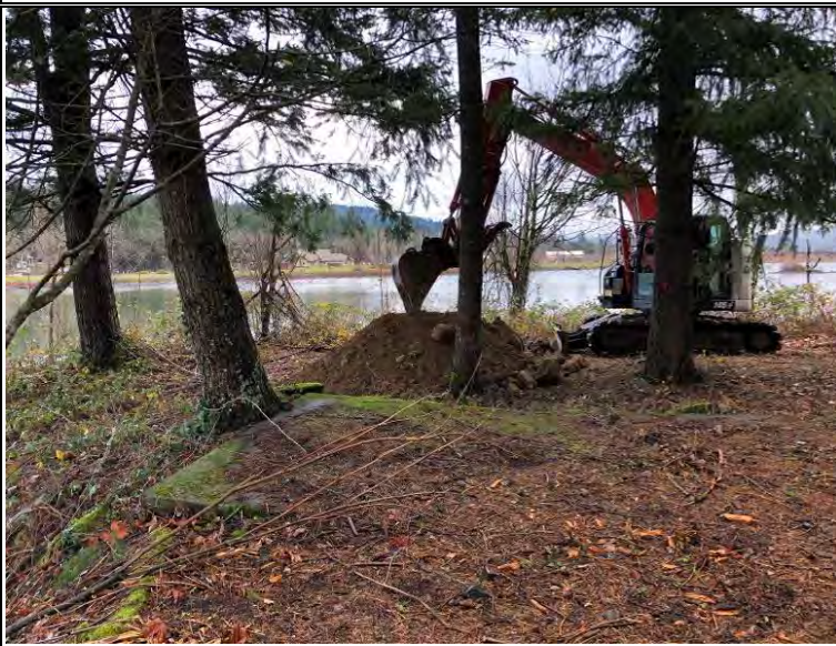
Excavation of test-pit TP-5, looking east
