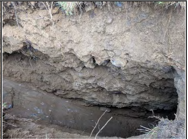
View of site conditions
