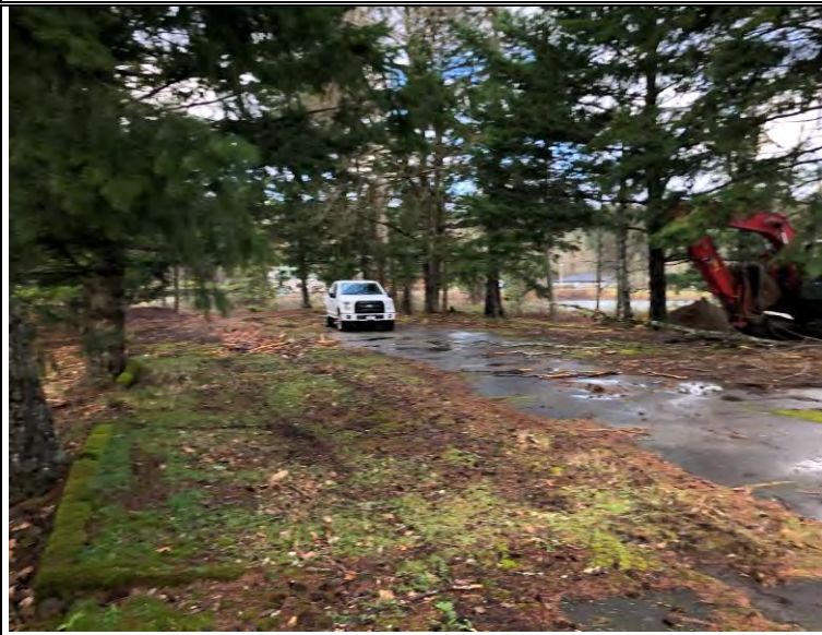
Excavation of test-pit TP-6, looking north
