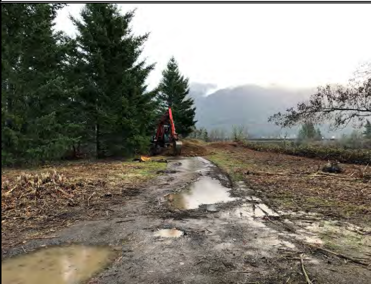
Excavation of test-pit TP-12, looking southwest
