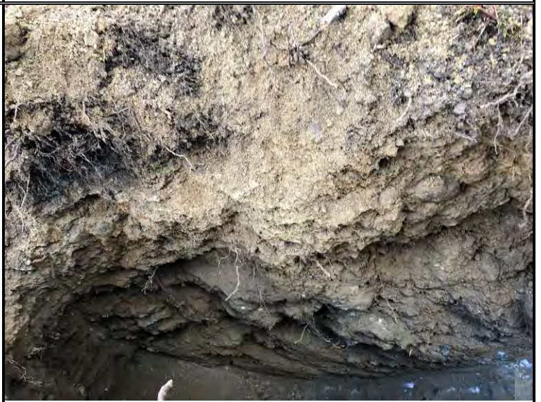
Exposed subsurface soil profile within test-pit TP-5
