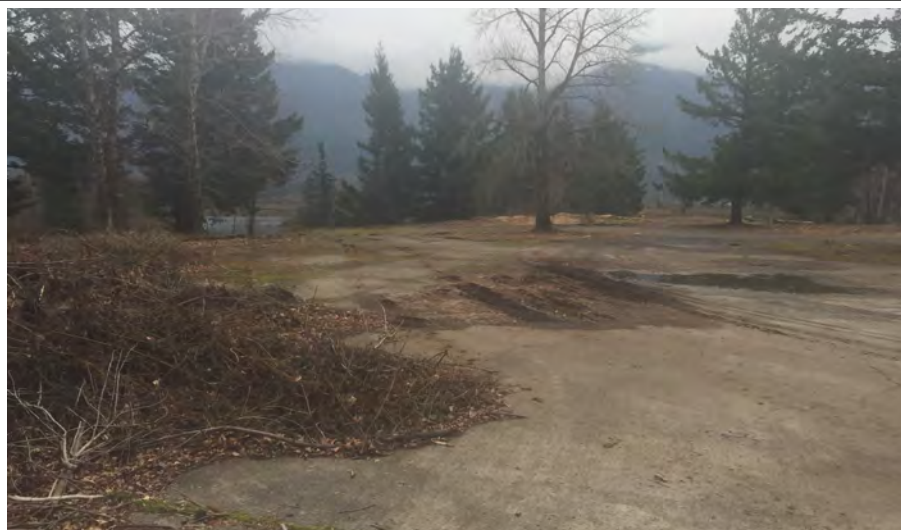
Photo 1. Existing concrete and gravel surfacing.
