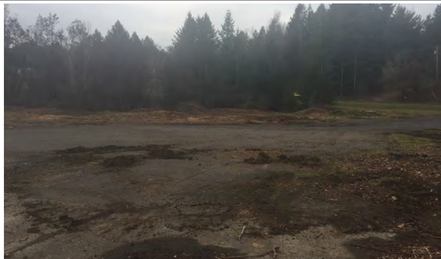
Photo 2. Existing concrete and gravel surfacing.
