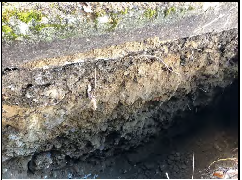
Exposed subsurface soil profile within test-pit TP-6
