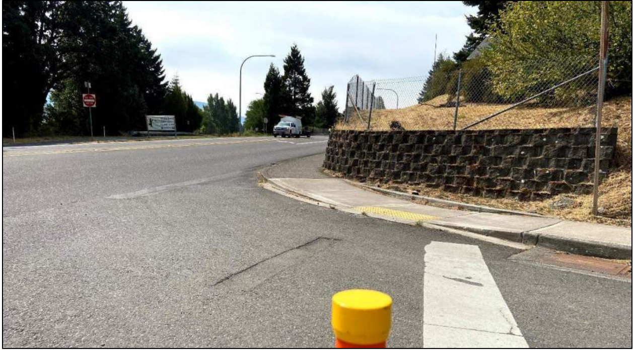
Lutheran Church Road at 2 nd Street Looking West
