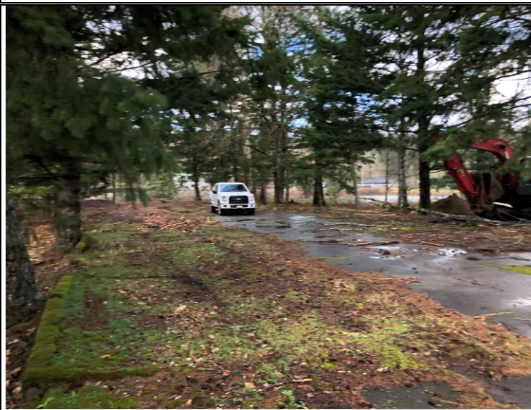
Excavation of test-pit TP-6, looking north
