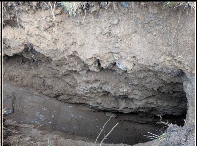
View of site conditions
