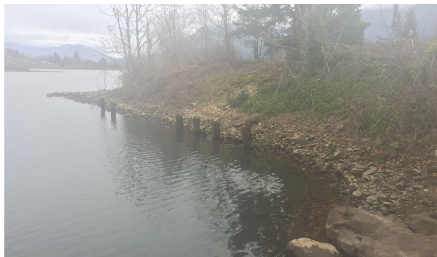
Photo 4. Riprap on the eastern shoreline, facing south.
