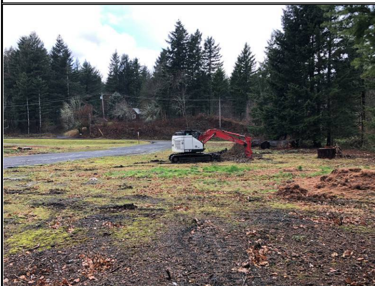
Excavation of test-pit TP-3, looking west
