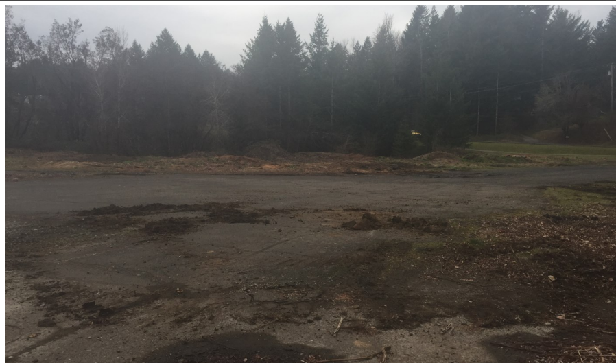
Photo 2. Existing concrete and gravel surfacing.
