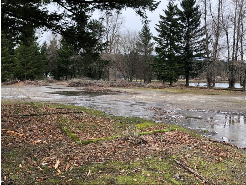
Figure 3. Photographic overview looking east at the concrete foundation of the main sawmill building of the HVM.
