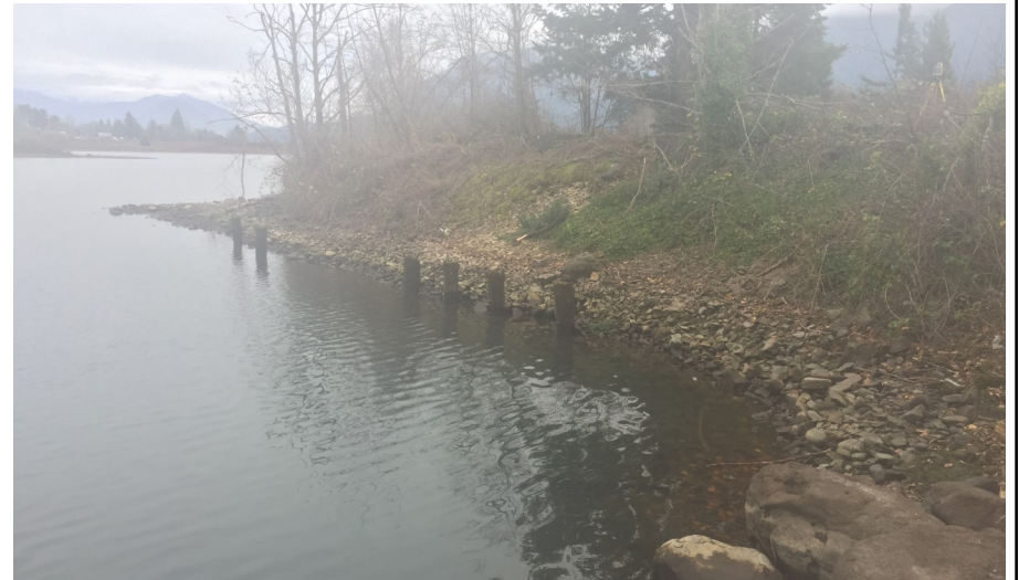
Photo 4. Riprap on the eastern shoreline, facing south.
