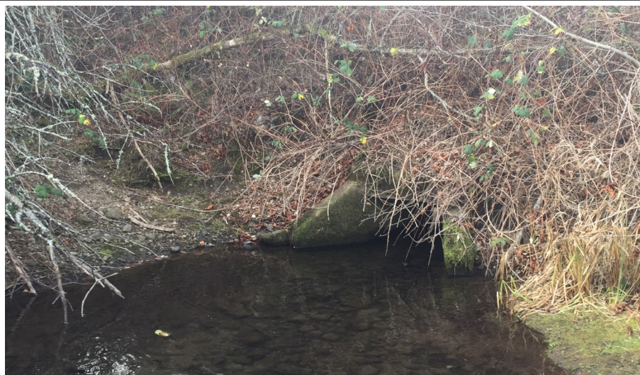
Photo 1. Inflow point of the unnamed tributary via concrete culvert.
