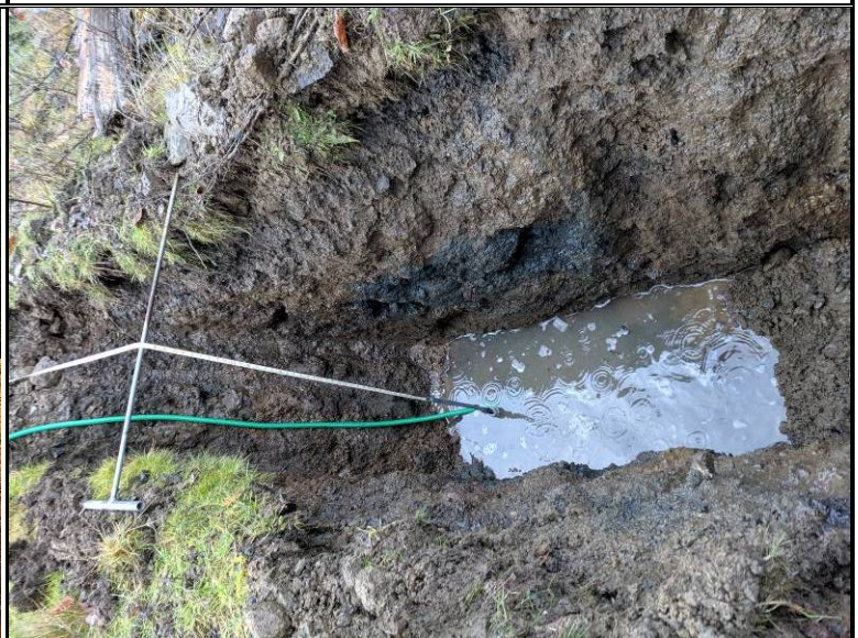
Infiltration test setup at test-pit P-1
