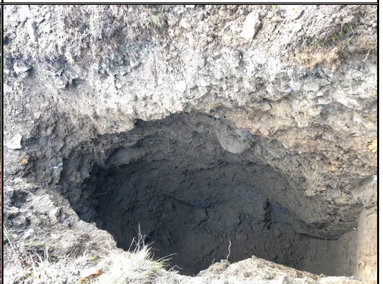
Exposed subsurface soil profile within test-pit TP-3
