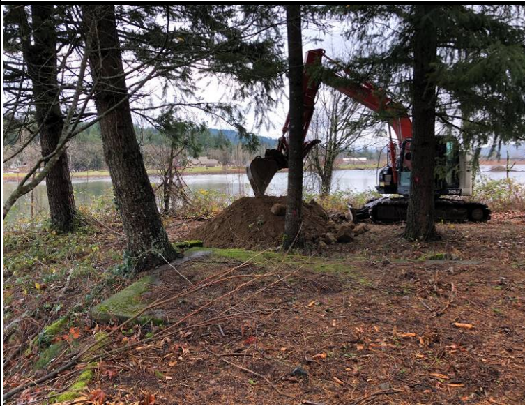
Excavation of test-pit TP-5, looking east
