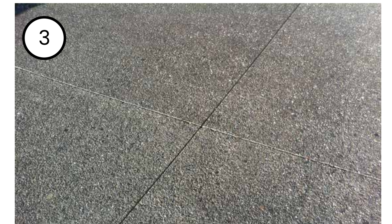
Concrete Paving with Exposed Aggregate Finish
