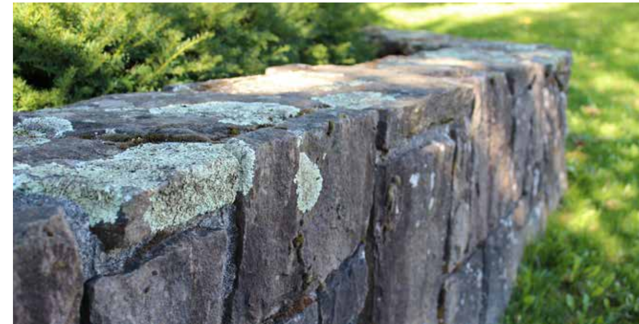
Basalt Ledge Stone Retaining Walls
