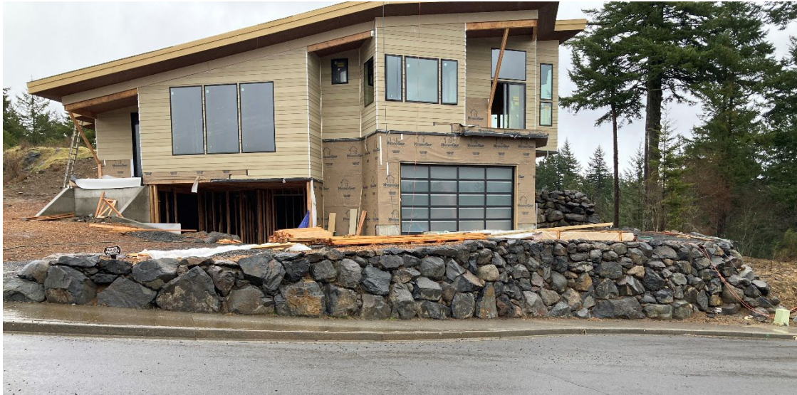
Figure 2 – 725 Angel Heights Rock Wall Looking East
