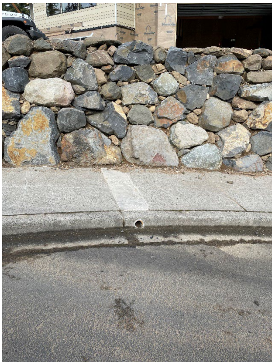
Figure 5 - Sidewalk Cut for Wall Drain
