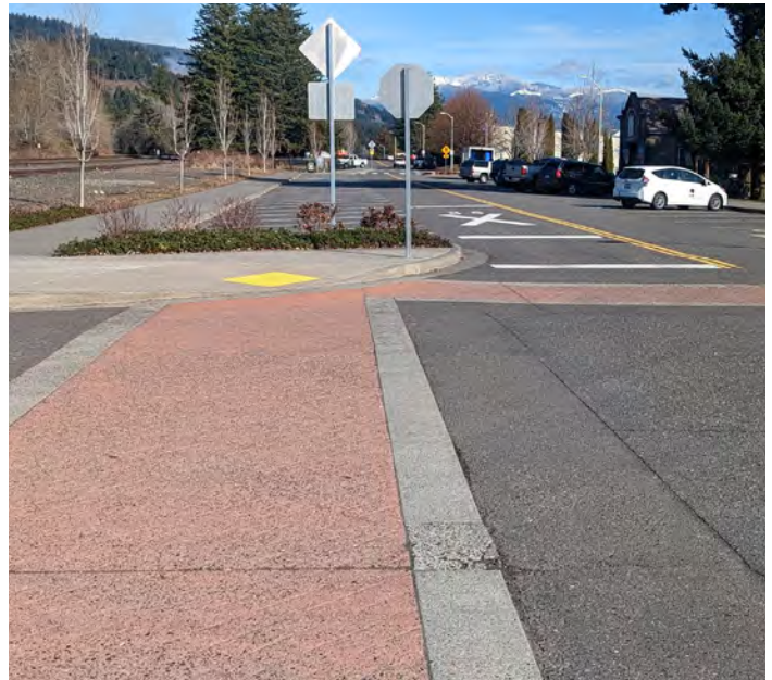
Existing crosswalk improvements for pedestrians.
