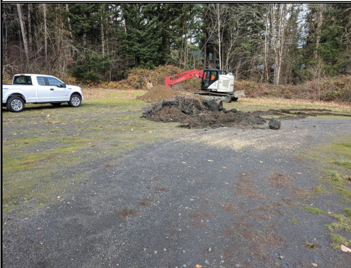
Excavation of test-pit TP-4 looking north
