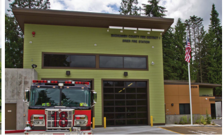
A5 Snohomish County Fire Station 18 - TCA
