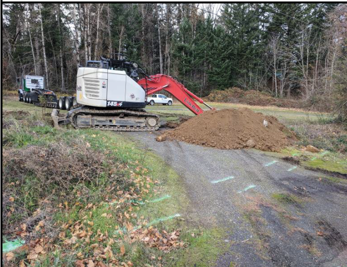
Excavation of test-pit TP-2 looking south
