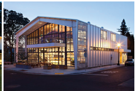
SHED - Jensen Architects B8
