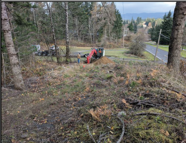
Excavation of test-pit TP-1 looking north
