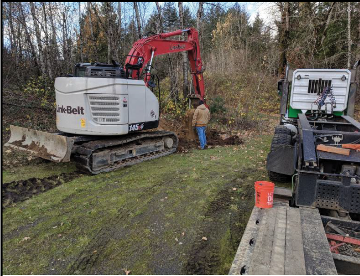
Excavation of test-pit TP-3 looking west
