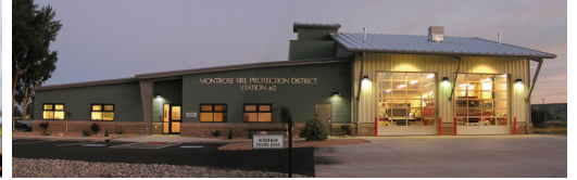
Montrose Fire Protection District Station 2 B6
