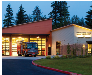
Snohomish County Fire Station 21 - TCA B7
