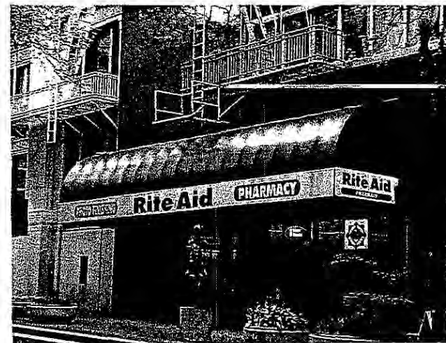
Inappropriate: Vinyl awnings
