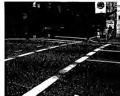
Not Appropriate: Single stripes wear out in heavy traffic and only minimally define the pedestrian zone
