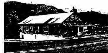
Appropriate: One-story wood frame building
