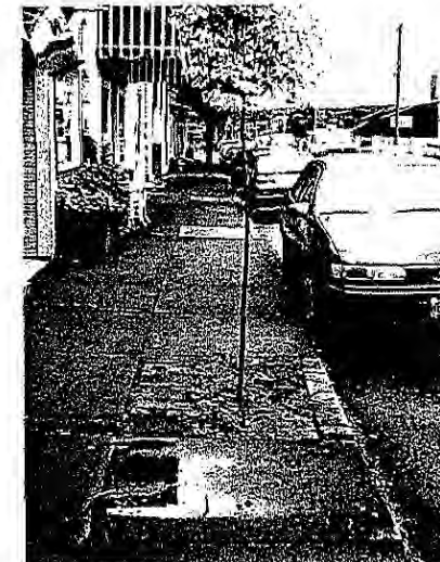
Not Appropriate: Narrow sidewalk without an adequate area for street trees
