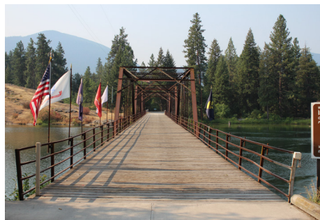
▲ Gallatin Bridge Over the Clark Fork
