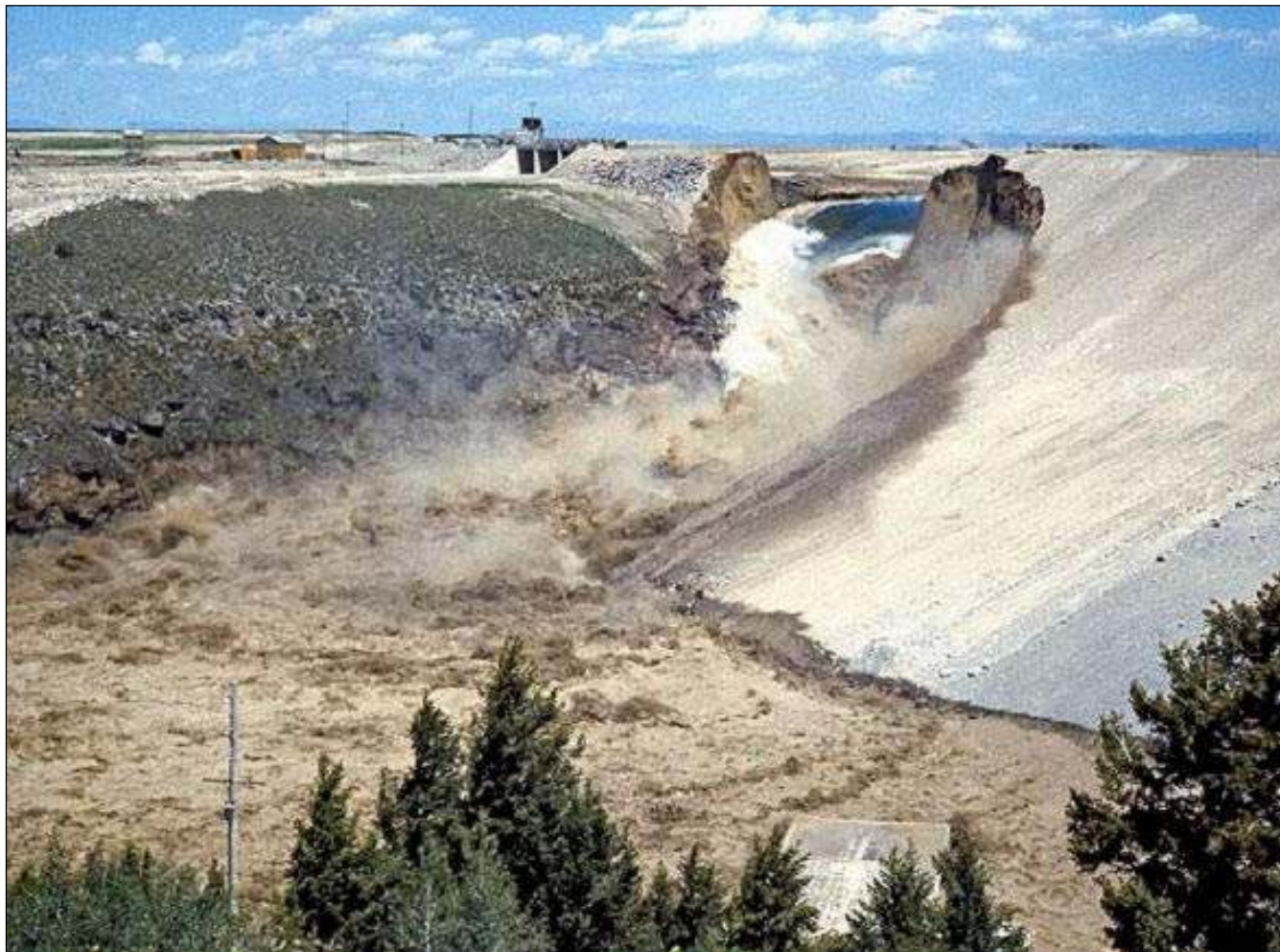
Figure 10-1. Teton Dam Failure, 1976
